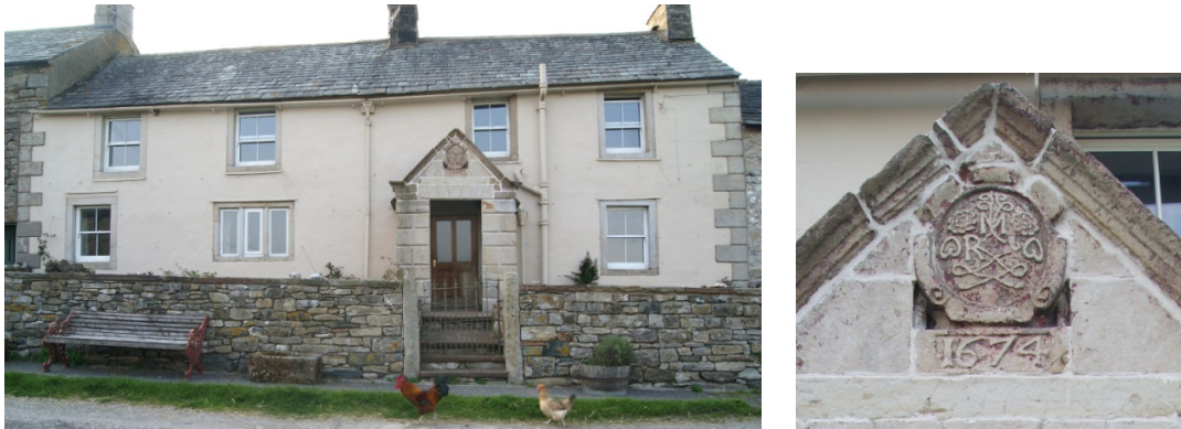
Figure 2. Widewath Farm: (a) general view, (b) porch with date stone
