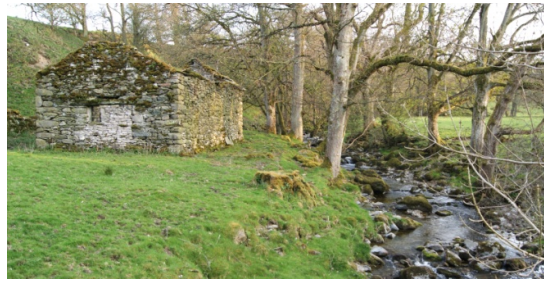
Figure 9. 'Old Widewath' barn: looking south
