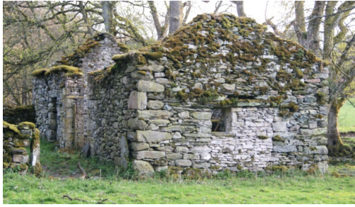
Figure 8. 'Old Widewath' barn: looking south-west
